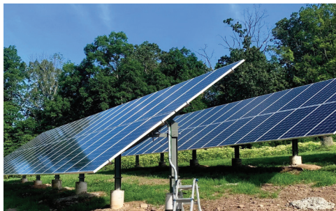
CONCRETE EMBEDDED POSTS
