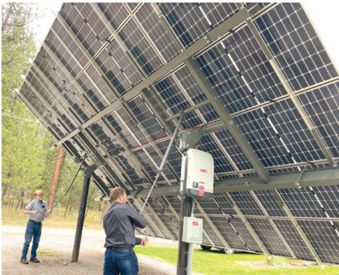
Tilt adjust system allows for seasonal tracking and access for cleaning.
