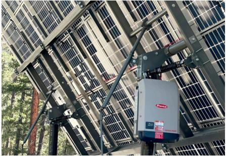
Adjust racking to desired tilt angle.
